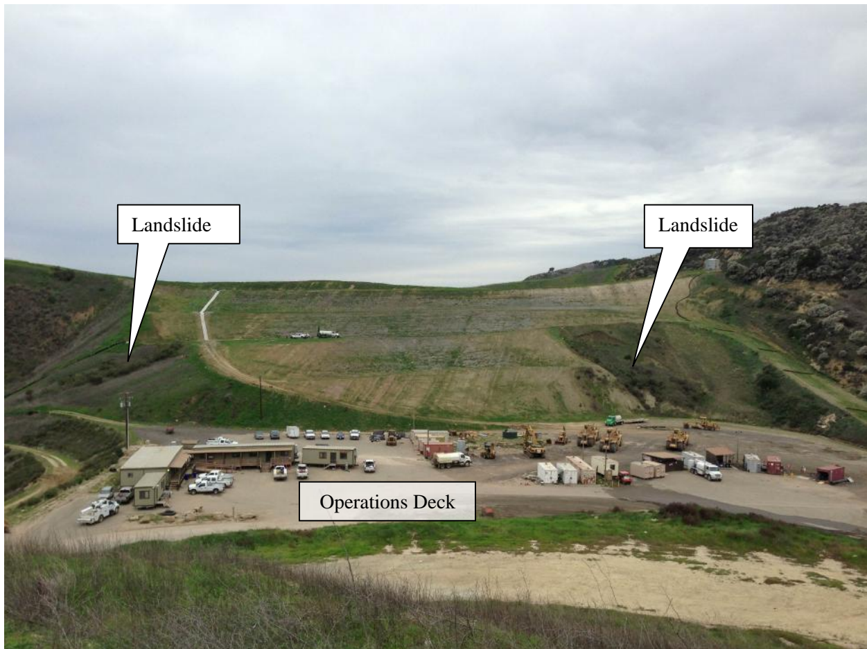
Figure 4: Photograph of the West Borrow Slope
