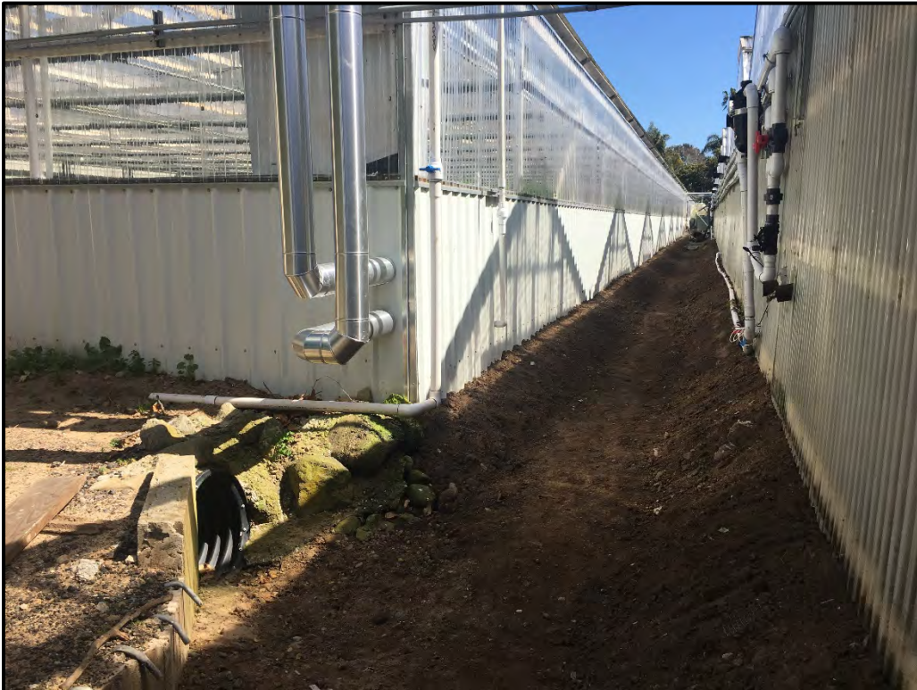
Photo 8: Culvert behind the water tank that discharges stormwater into Arroyo Paredon Creek (Aspect: East).
