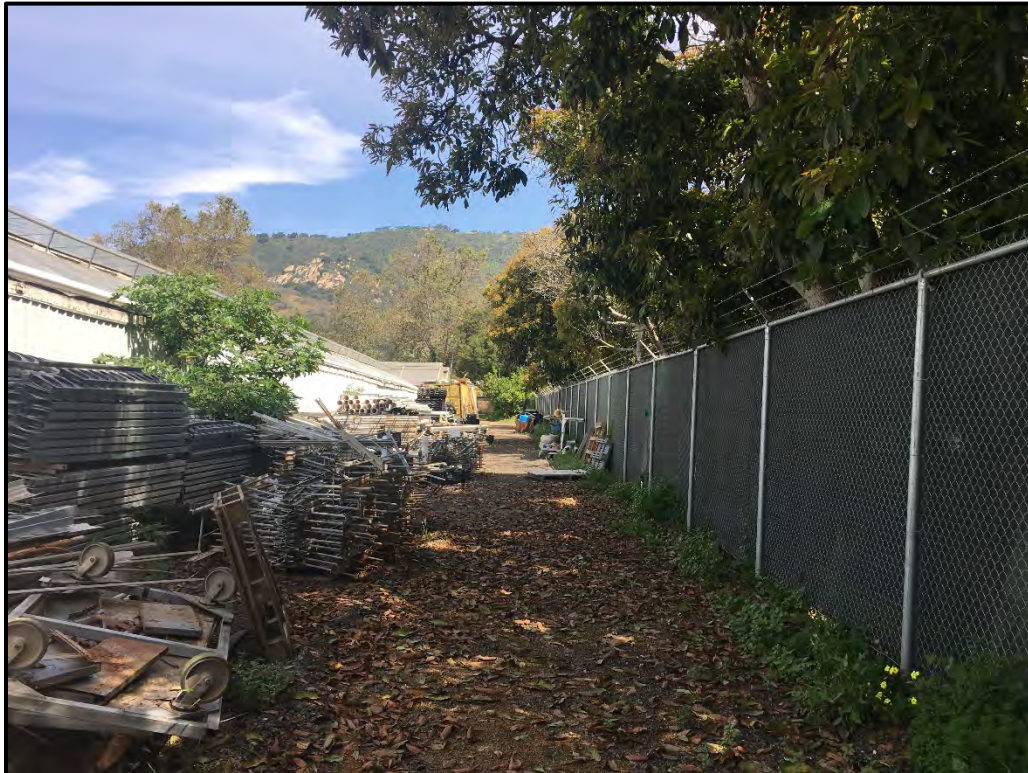
Photo 4: East side of Project Site where underground stormwater detention basin will be located, outside of the ESH buffer (Aspect: North). Photo taken 5/7/2020.
