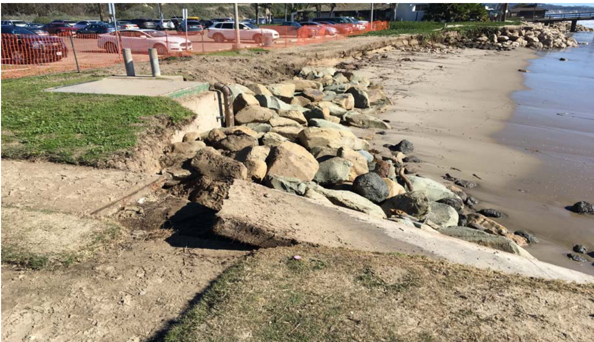
Photograph 2. Rock Revetment Protection for Outfall Access Vault
