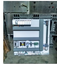
SCS RMC panel prior to installation
