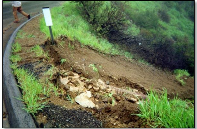
Gibraltar Road at MP 3.1 looking southeast
