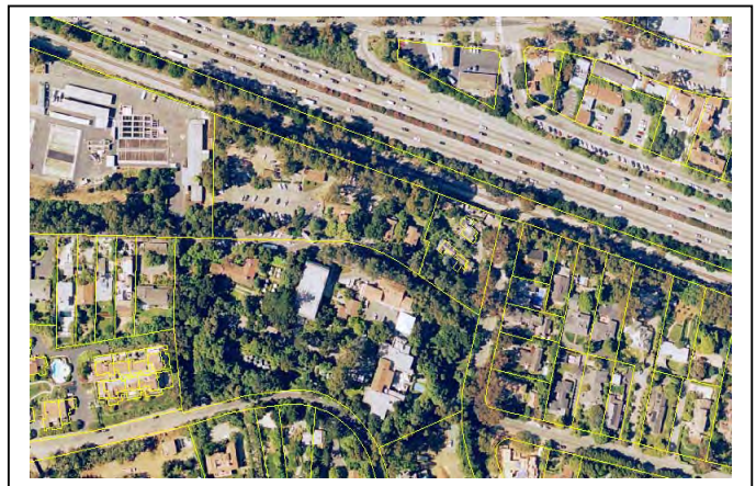
Assessor Parcel Numbers 9-282-029, 030. The project site is located immediately south of the Union Pacific Railroad tracks and Highway 101, between Butterfly Lane and the Montecito Sanitary District facilities, commonly known as 1070 Fairway Road (also referred to as "The Fairway"), in the Montecito area, First Supervisorial District.
