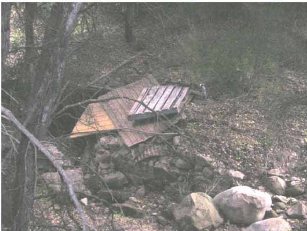
Hand-dug well with an opening of approximately five or six feet across and an unknown depth
