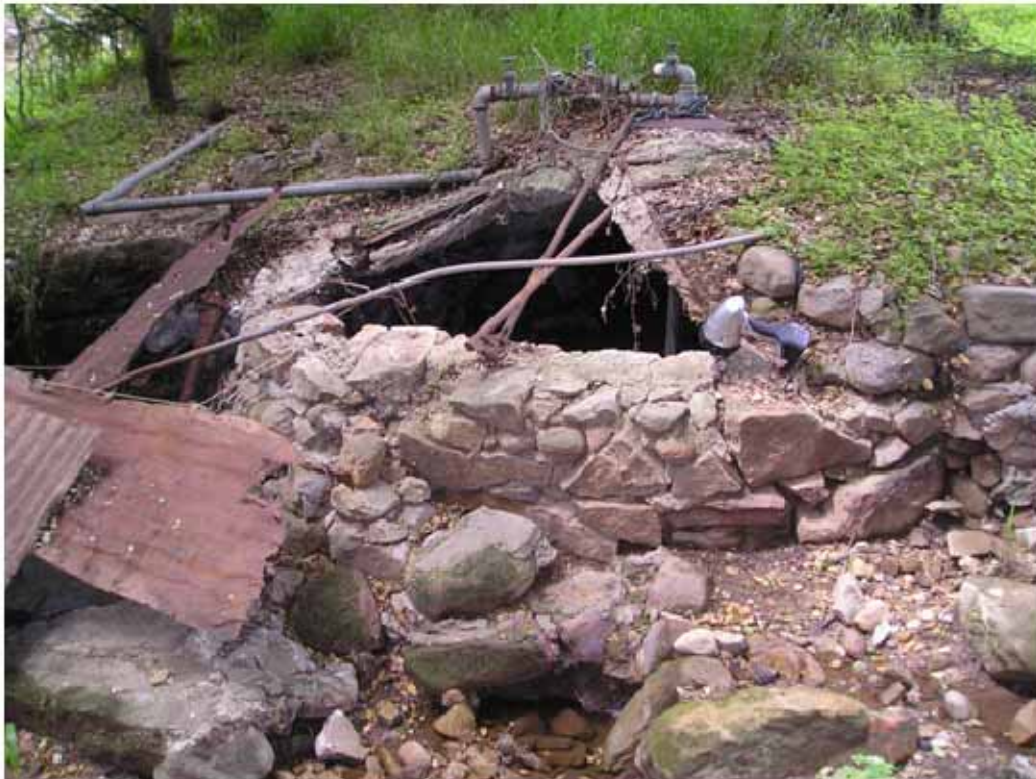
Hand-dug well with an opening of approximately five or six feet across and an unknown depth
