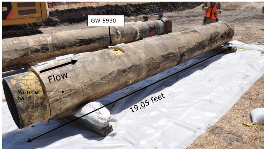
Figure 2. Photograph showing Pipe Section 1 following removal from the ditch.
