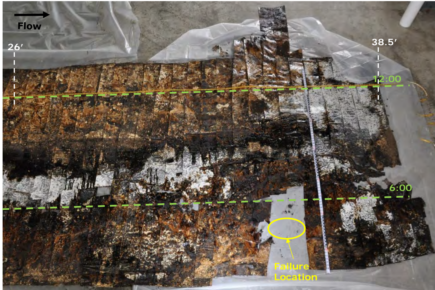
Figure 12. Photograph showing the internal surface of the external tape at the failure location. Tape measure indicates distance to upstream girth weld.
