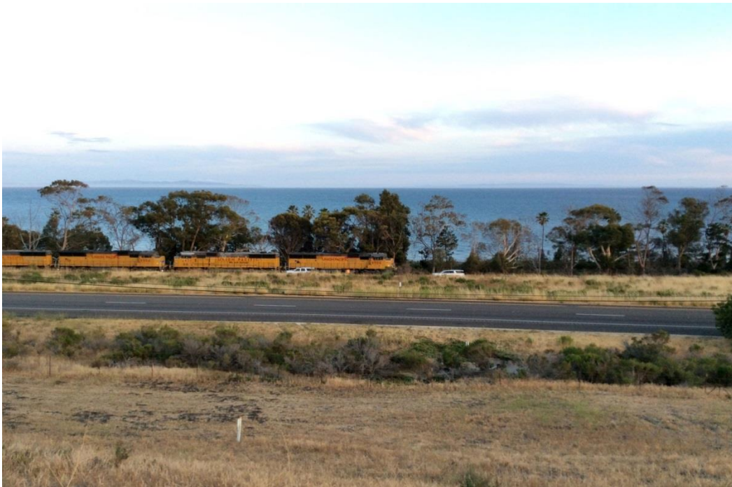
Culvert Under Highway and RR Tracks to Ocean
