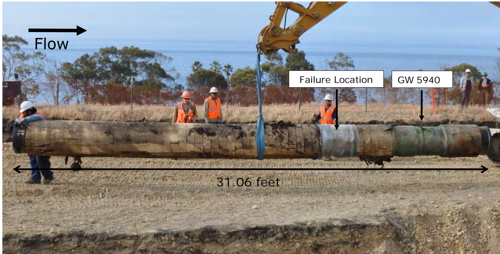
Figure 3. Photograph showing Pipe Section 2 being removed from the ditch.
