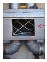
Autopsy Lab Exhaust Duct Filter. Requires Regular Replacement.
