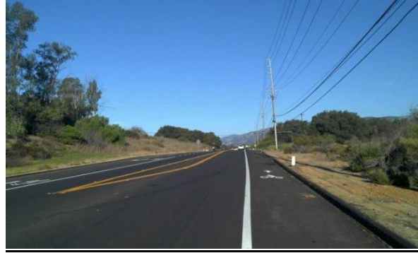
After: section of Cathedral Oaks Road
