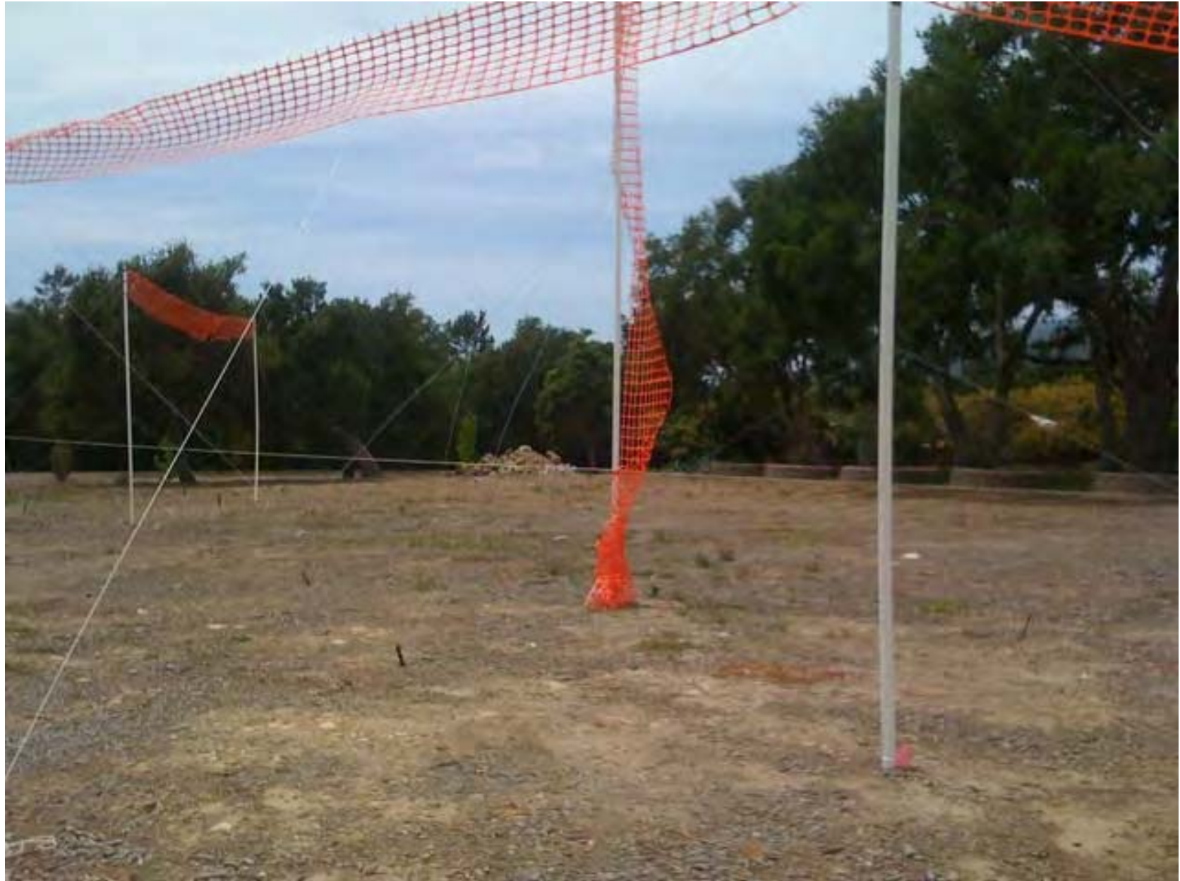
Applicant Story Poles Showing Finished Floor
