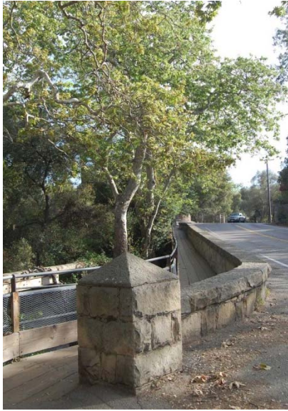
Historic Stone Bridge
