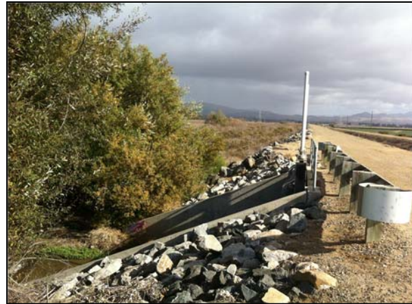
Photo of the existing channel at the northern-most portion of the Project site. Santa Maria River to the left, Santa Maria River Levee Road to the right and agricultural field to the far right.
