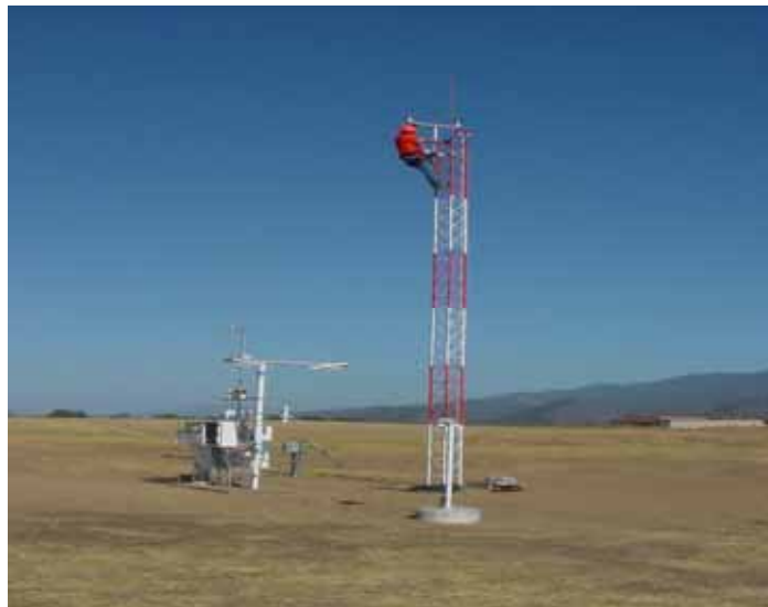
Photo: Completed AWOS at Santa Ynez Valley Airport
