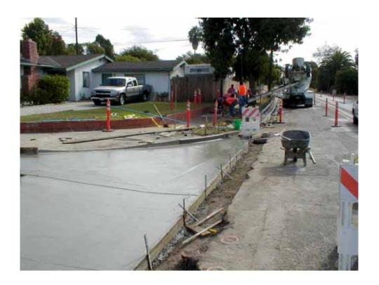
The project is one of the strategies the Department employs in its annual Preventive Maintenance Program and consists of the repair of the existing hardscape by the removal and replacement of damaged concrete curbs, gutters and sidewalks, installation of federally mandated curb ramps, tree root pruning and shielding. Approximately 753 linear feet of sidewalk and 895 linear feet of curb and gutter will be repaired with the construction of this project.
