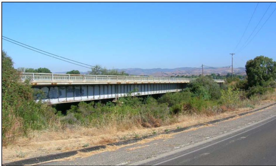
Existing Bridge No. 51C-173on Santa Rosa Road
