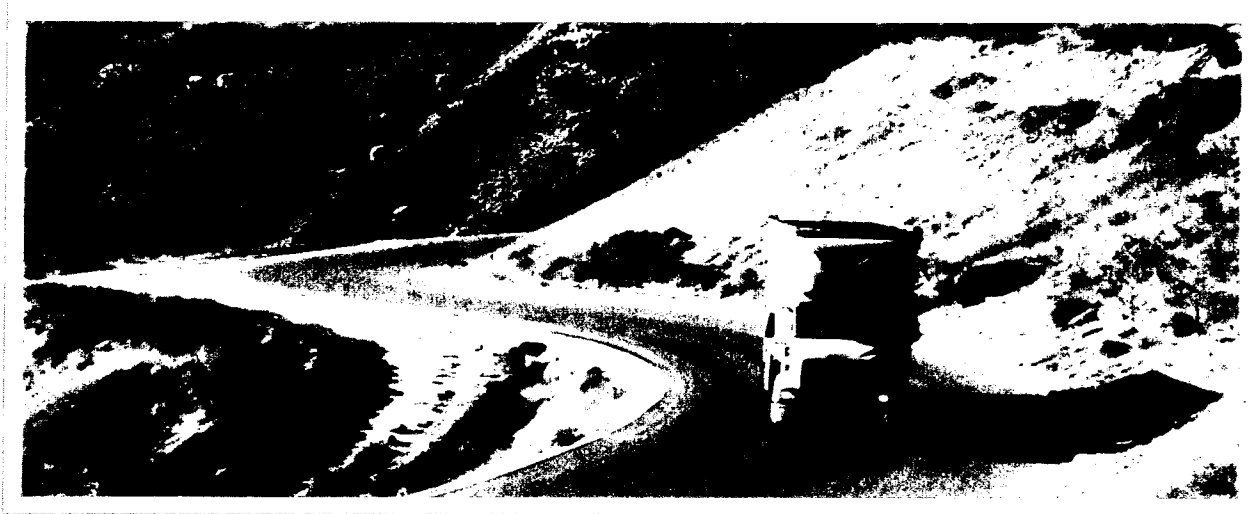
Tajiguas Landfill: Bengal designed specialized roadways for heavy traffic in steep country.
