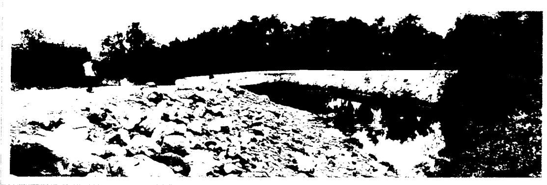
View looking south along the approximate alignment for the proposed HDPE By-Pass Pipe. Note Rock Slope Protection which covers the ground here.
