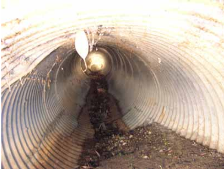
Existing Pipe Culvert under Alston Road
