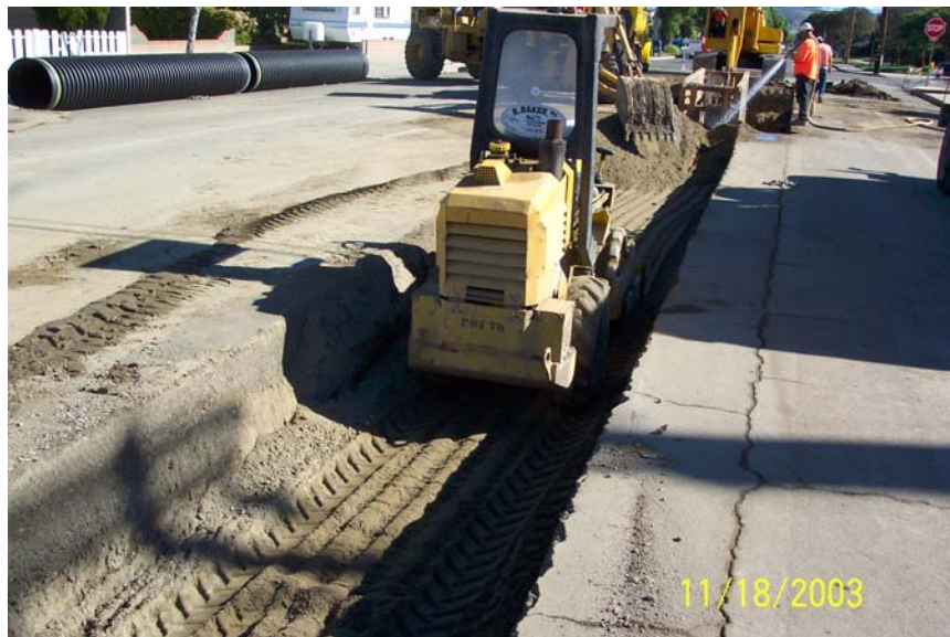
Construction of the College-Walnut Storm Drain Laterals Project
