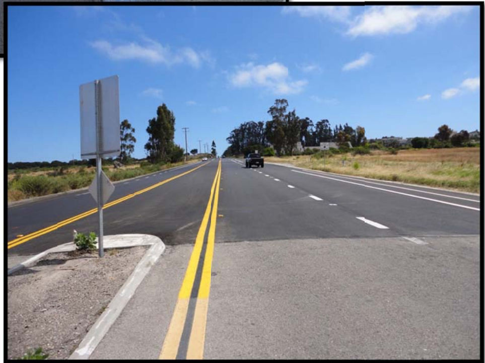
Completed Harris Grade intersection at Highway 1
