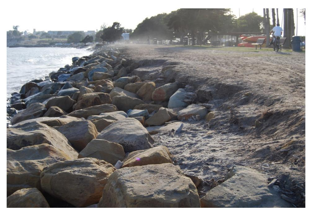
Goleta Beach Park eroding behind the new emergency revetment during mild summer wave conditions. \$950,000! Doesn't work, destroys the beach.
