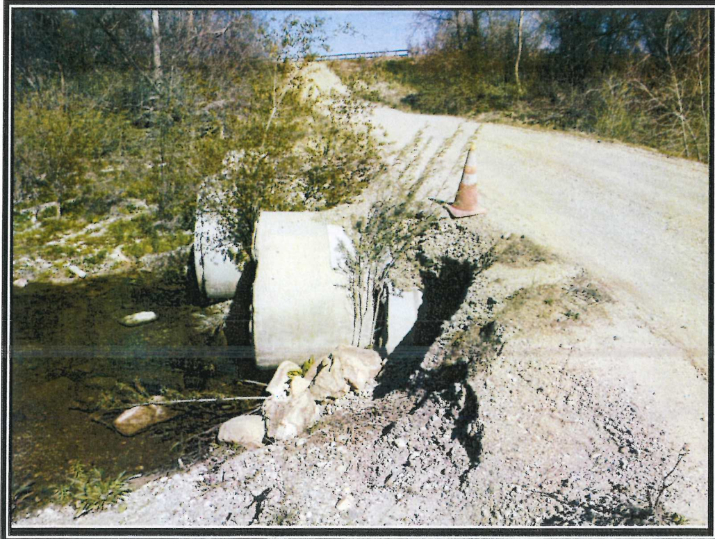
Looking North at Arizona Crossing (#788)
