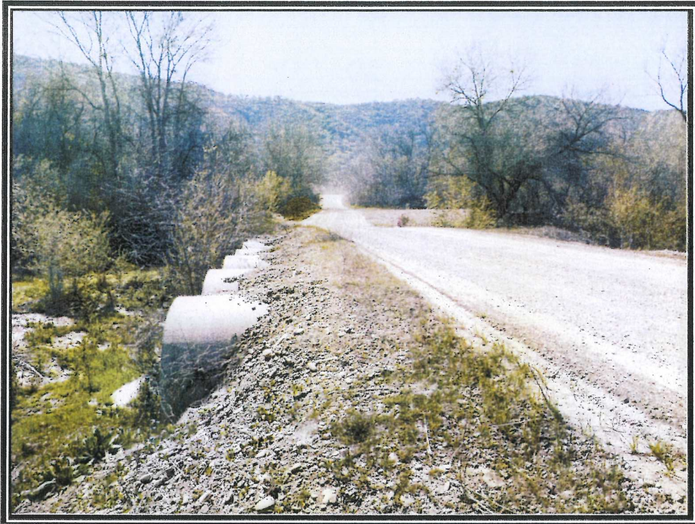
Looking South at Arizona Crossing (#784)
