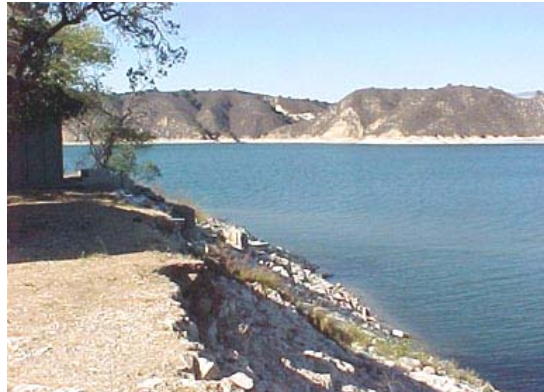
Current low lake level conditions at Water Treatment Plant
