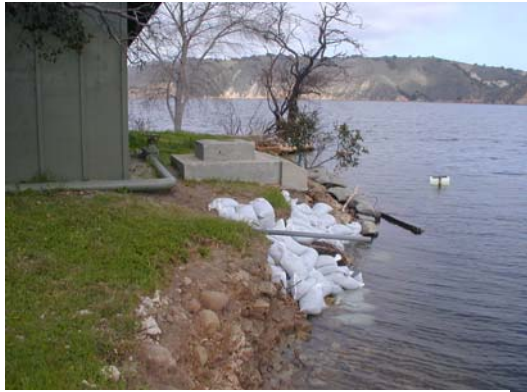
March 2001 photo of lake embankment adjacent to Water Treatment Plant
