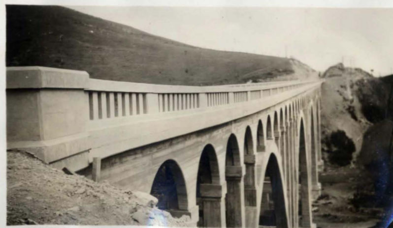
Railing Constructed on Vertical Curve. S. B. Z. F. Cont. #229 -
