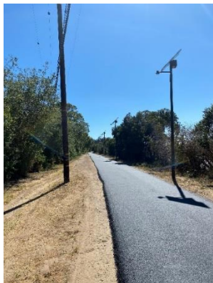
Obern Trail Rehabilitation
