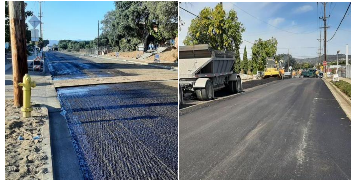
Rucker Road – Grind, overlay, and dip reduction
