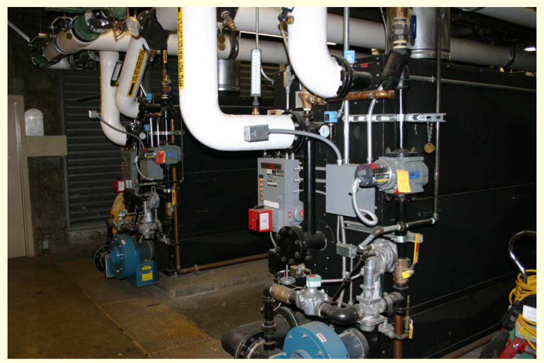
Boiler Replacement Project
