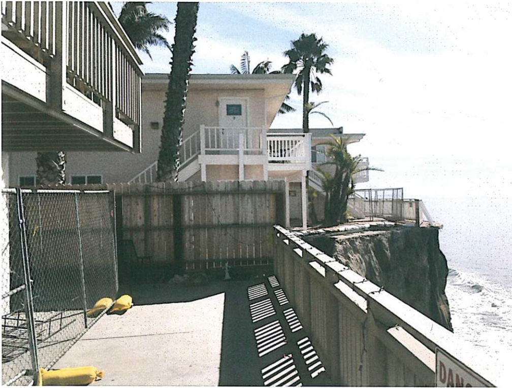
LOOKING EAST FROM SOUTHWEST CORNER OF REAR PATIO
