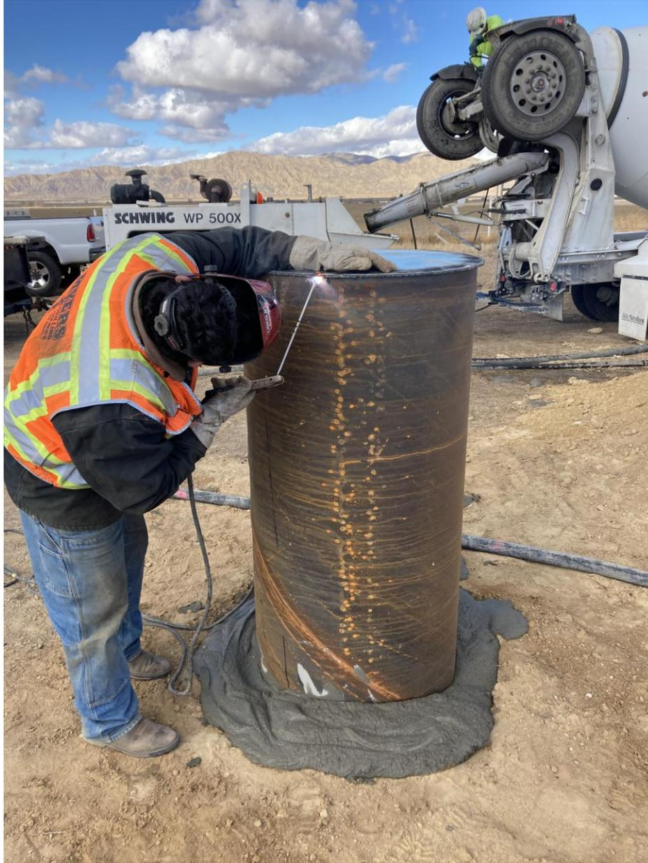
***Welding 32" steel cap on top of 30" steel casing
