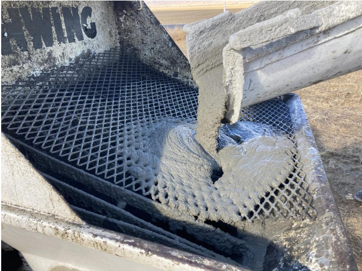
*Pouring cement into pumper hopper
