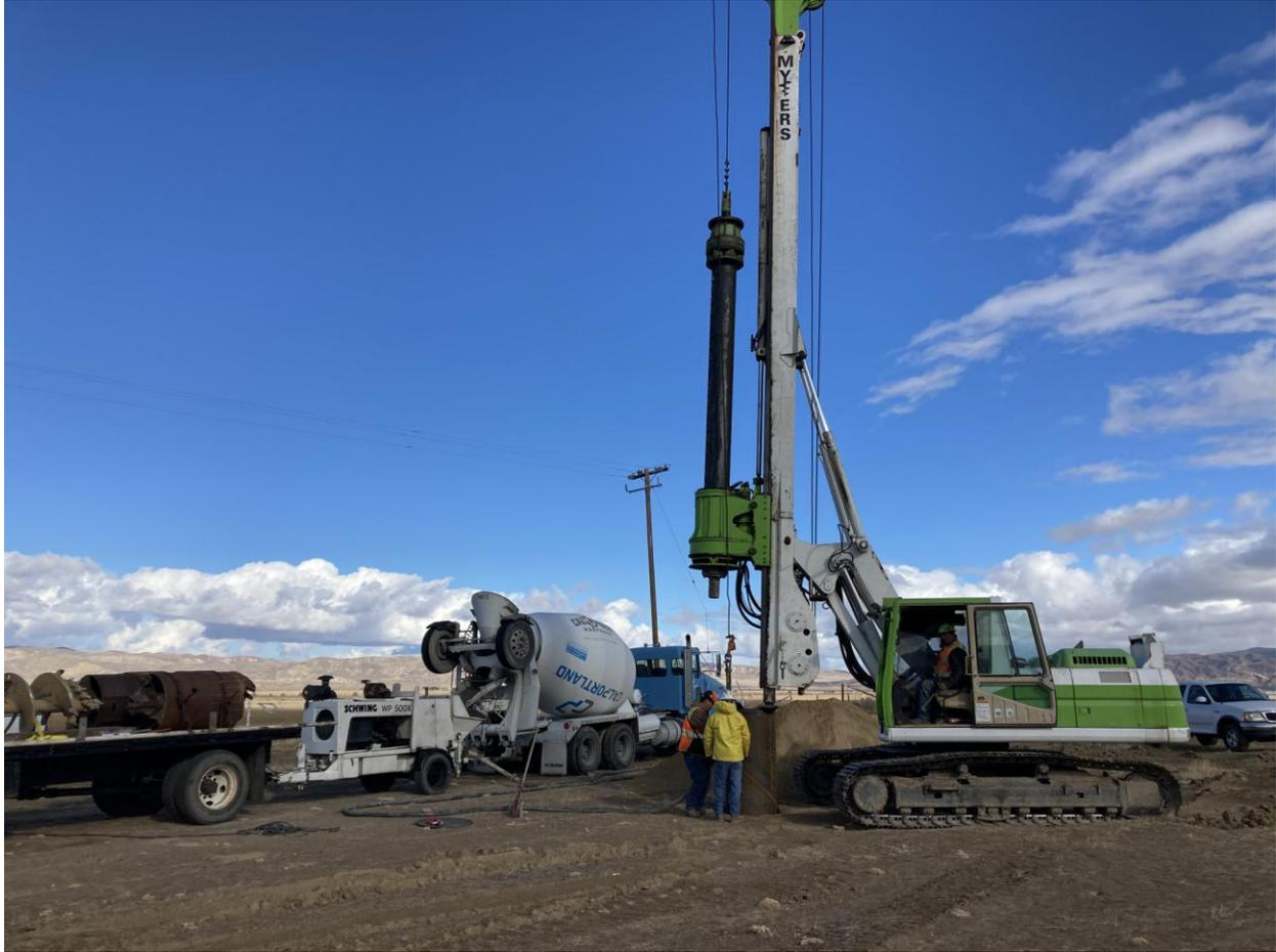
*Myers Brothers Drill Rig, casing installed, pumper and cement truck
