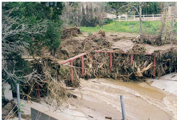
Figure 2 – Existing Debris Rack on Tecolote Creek during the 1998 Floods
