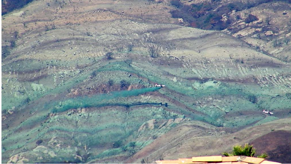
Figure 4 – Aerial Hydromulching (Gap Fire 2008)
