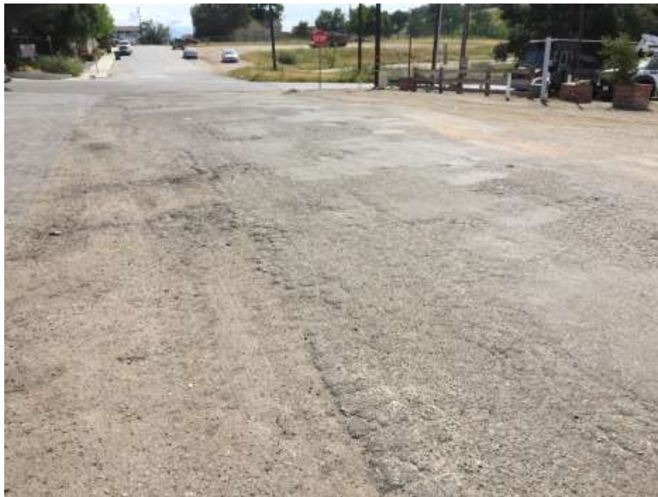
Example road to be rehabilitated – Numancia Street
