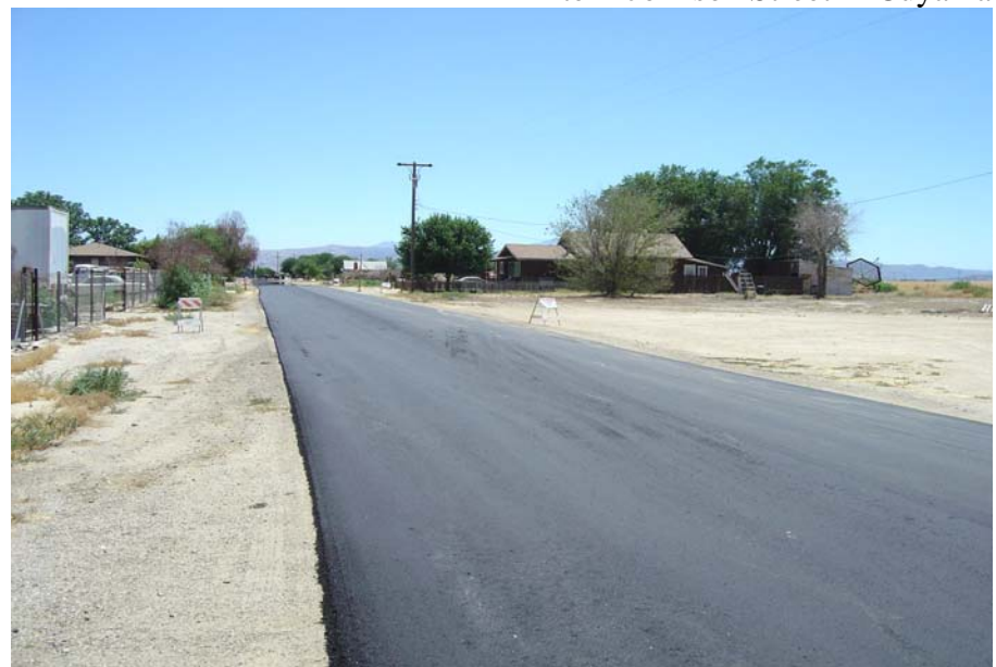
After - Johnson Street in Cuyama
