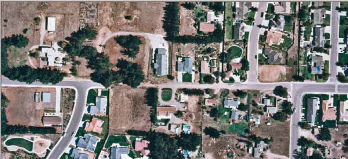
Photo of unimproved section of Hummel Drive
