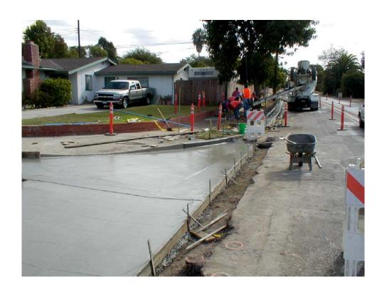
The project is one of the strategies the Department employs in its annual Preventive Maintenance Program and consists of the repair of the existing hardscape by the removal and replacement of damaged concrete curbs, gutters and sidewalks, installation of federally mandated curb ramps, tree root pruning and shielding. Approximately 3,534 linear feet of sidewalk and 3,437 linear feet of curb and gutter will be repaired with the construction of this project.
