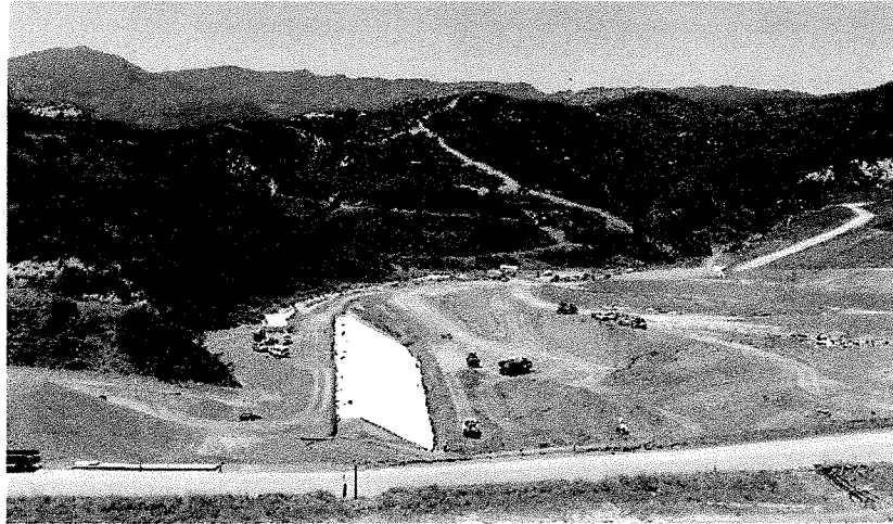
Geomembrane placed along an engineered fill berm during construction of Phase IIIC.
