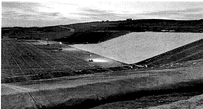
CQA during liner installation at Taft Landfill.
