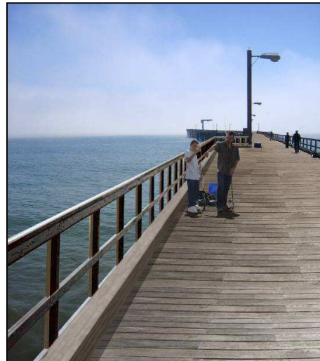
Deck over new pilings
