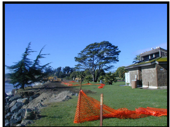
Park Erosion at Existing Restroom – 2002
