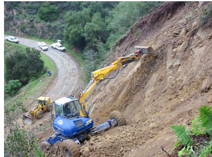
Landslide repair on Stagecoach Road
