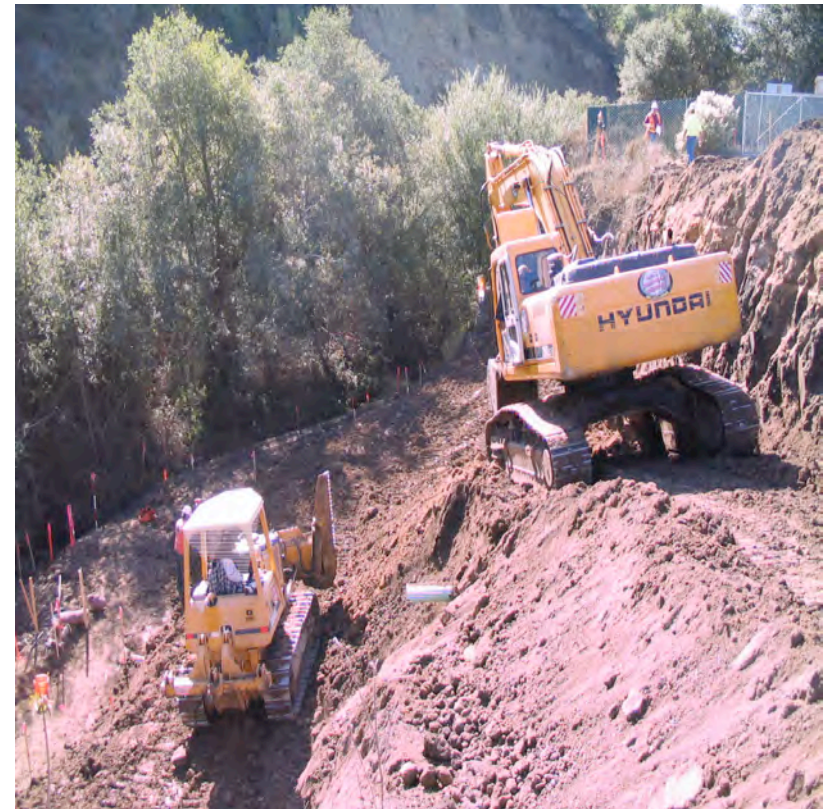
Bank Stabilization/Landside Repair
