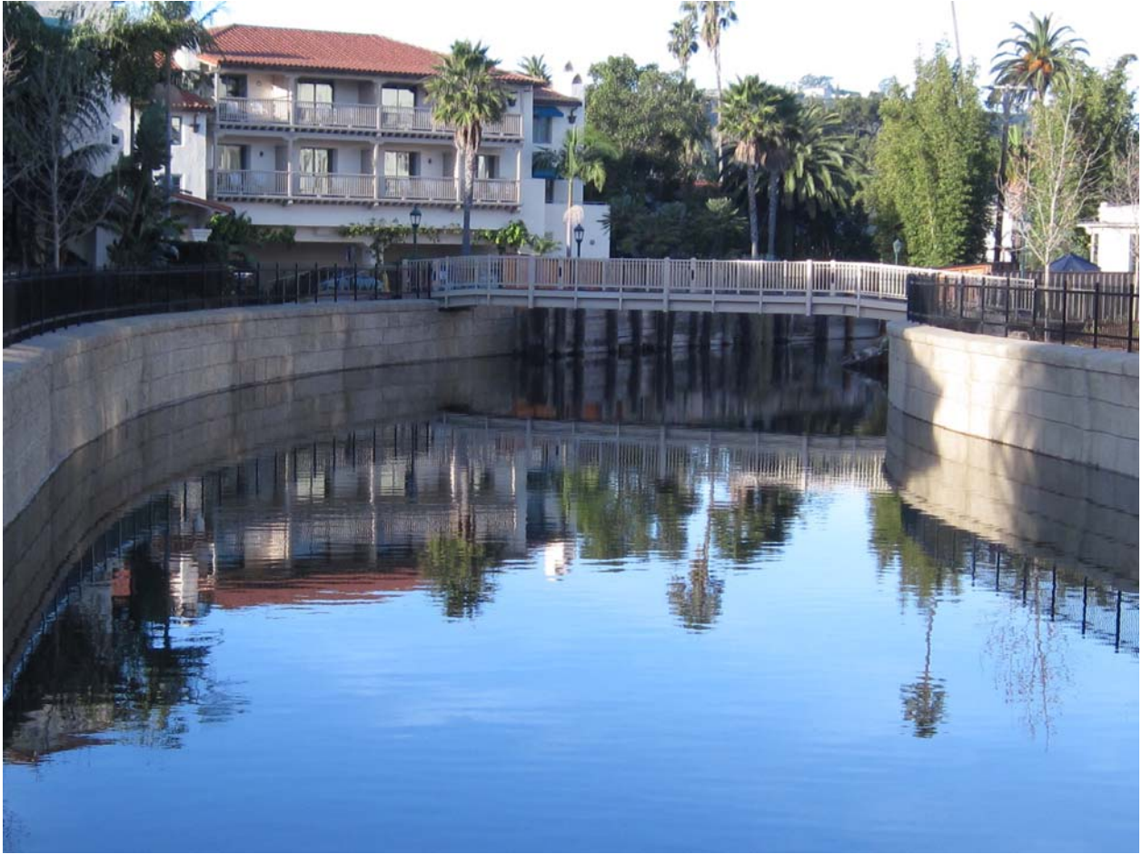
Lower Mission Creek 1A-1 Project Completion
