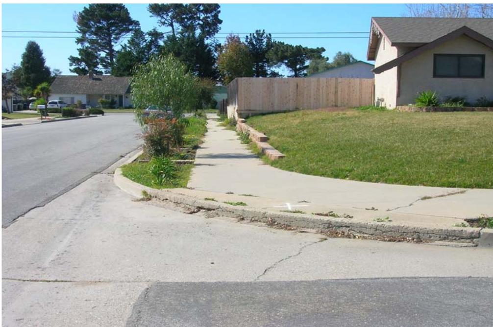
*Typical site for concrete repairs; at this site the spandrel will be repaired and a new ADA-compliant curb ramp will be constructed.*
