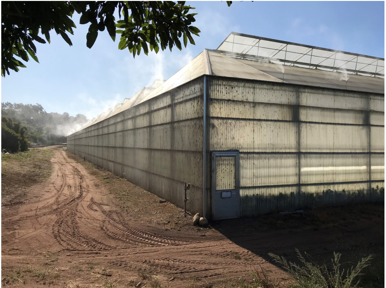
ODOR CONTROL ON NORTH SIDE OF THE GREENHOUSE AT VALLEY CREST FARMS
