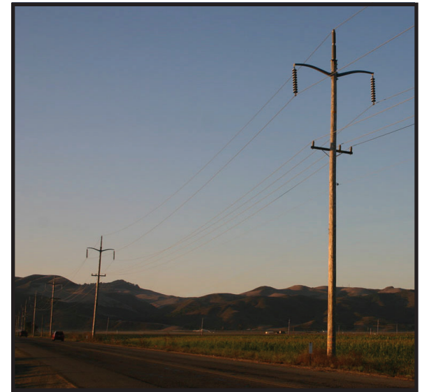
C Example of Typical Power Line Pole Structure
