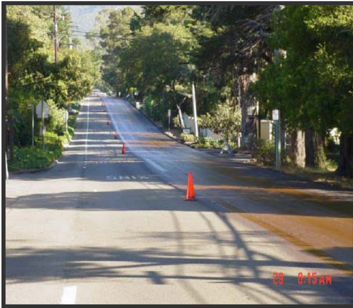
Figure 1: Fog seal applied to one lane.
