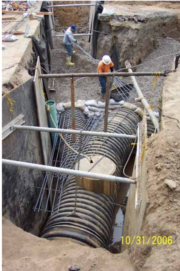
Construction of the Westside Storm Drain Project Phase II
