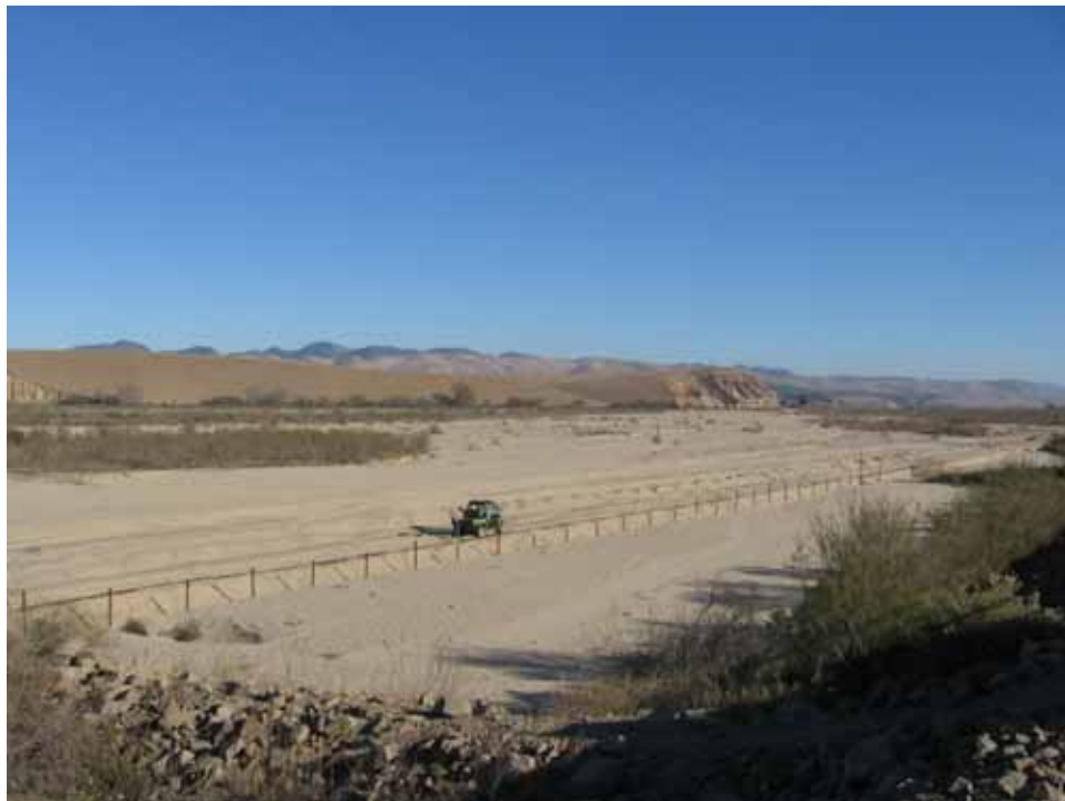
Pipe & Wire Work
