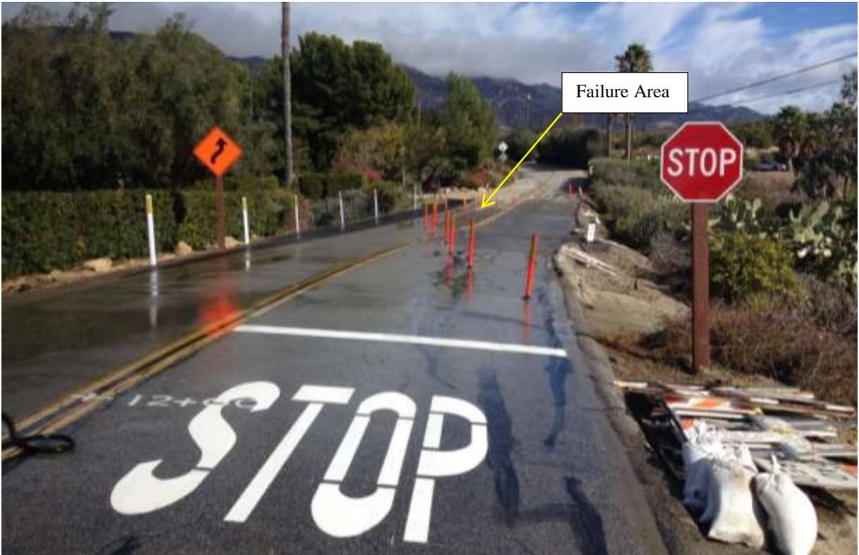
**View of Ortega Ridge Road, looking east, showing temporary traffic controls. Area of roadway that is delineated by orange channelizers continues to differentially settle, and has continued into left-hand lane.**
