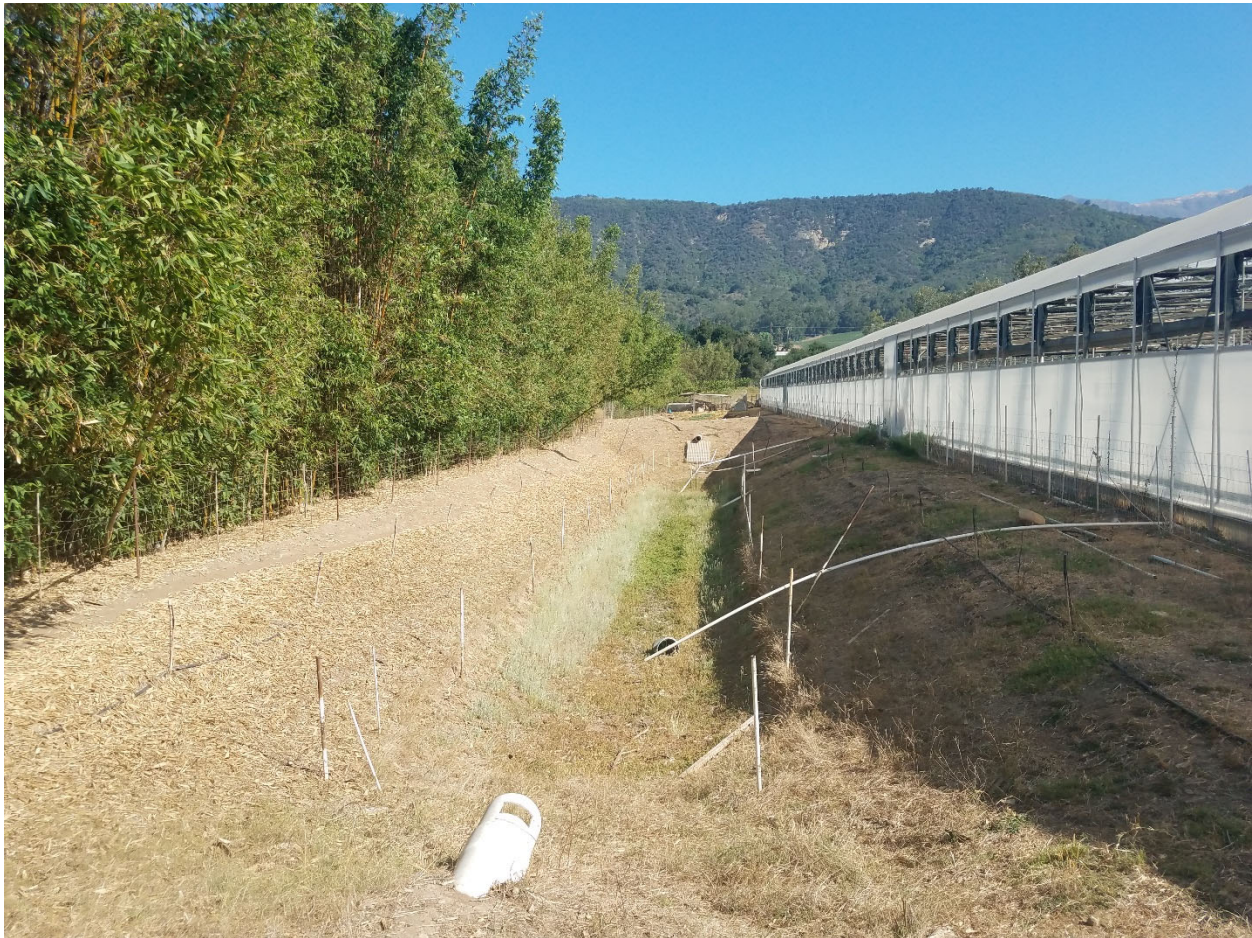
Figure 4- Typical Existing On-site Stormwater Retention Basin
