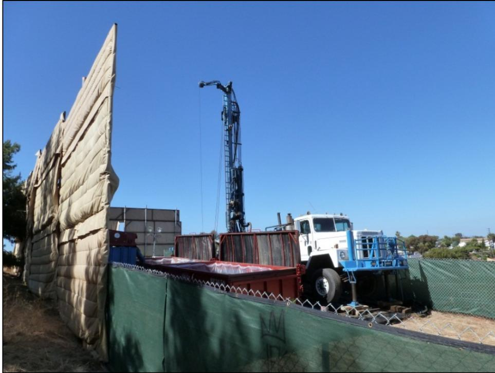
**Figure 17 – Sample Temporary Construction Noise Barrier (URS, 2012)**
