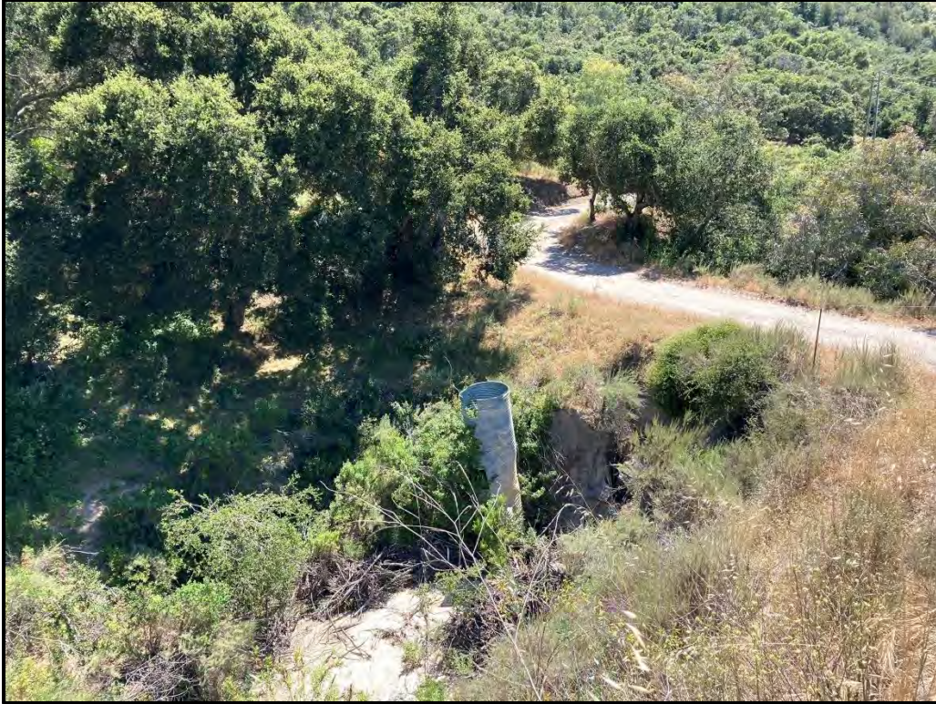
Photo 5 – Existing culvert at the entrance driveway (Aspect: South).
