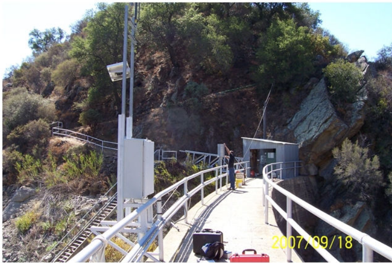
Water Level & Rain ALERT Instrumentation
