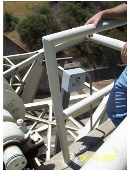
Dam Gate Inclinometers
