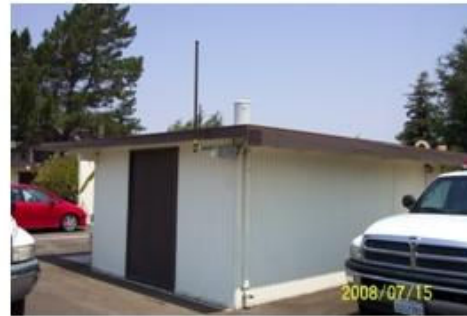
ALERT 0.01" Rooftop Install (Buellton Fire)
