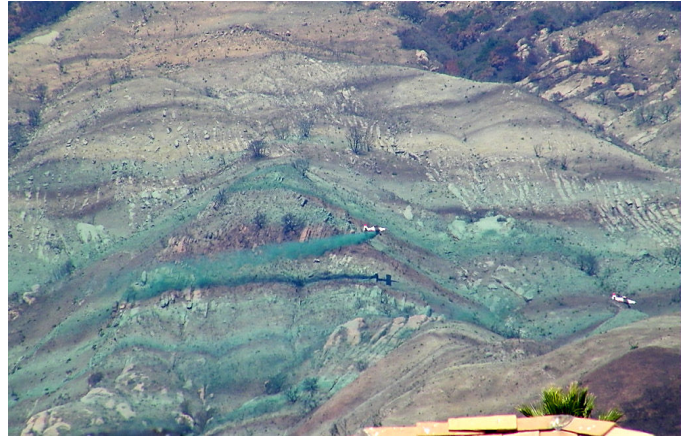
Figure 19 – GAP Aerial Hydro-mulching – Oct 2008
