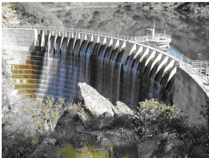
Figure 73 – Juncal Dam & Spillway
