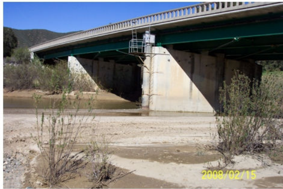
ALERT Shaft Encoder (Cuyama River @ Buckhorn)
