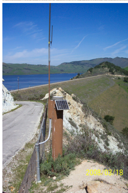
Figures 75 & 76 – Twitchell Reservoir & Dam
