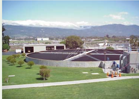
Goleta Sanitary District — Biofiltration Unit
