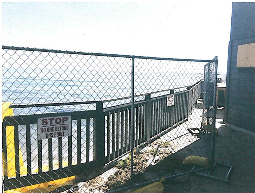
LOOKING SOUTHWEST FROM SOUTHEAST CORNER OF REAR PATIO
