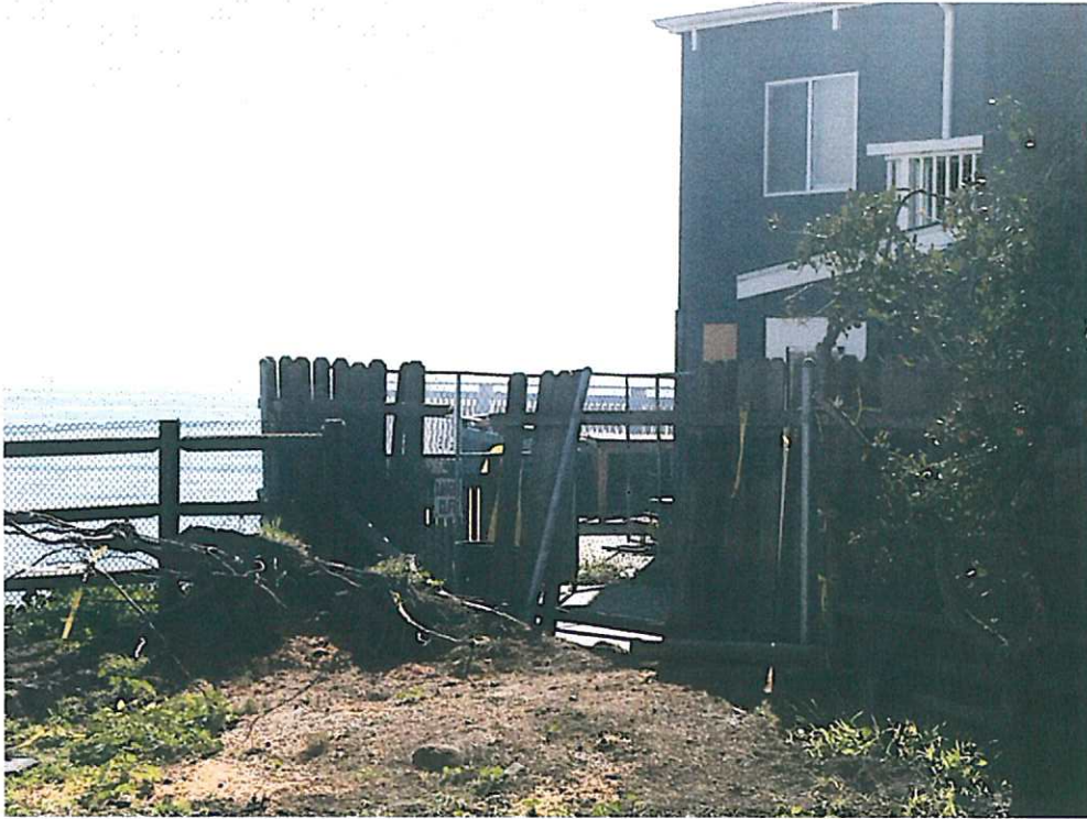
LOOKING SOUTHEAST TOWARD 6757 DEL PLAYA REAR PATIO FROM THE ADJACENT PARK
